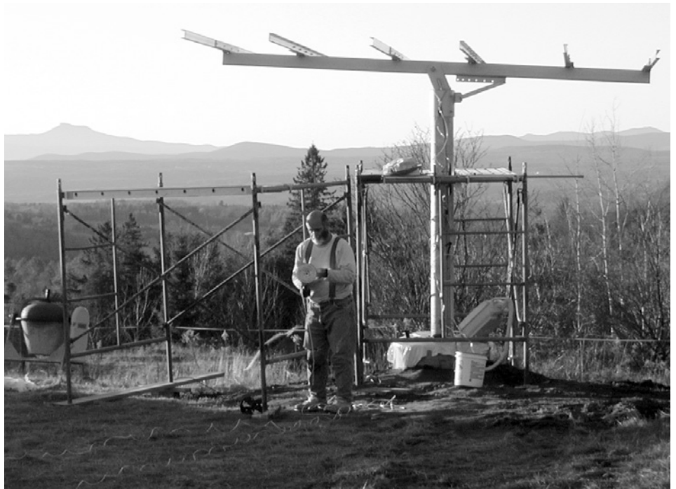
Ed Hutchinson installing and wiring one of the family's two 2,500-W, pole-mounted PV arrays (above and below). It's the two pole-mounted systems that are tied into the grid and, converted from DC to AC power, contribute to the Co-op's electricity network. Photos courtesy of Ed Hutchinson.
