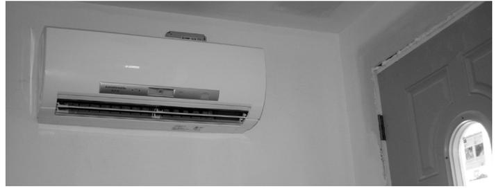
*Above: Just inside the doorway at the Waterbury house, a unit mounted on the wall uses air warmed and transferred from outside to boost the temperature of the indoor air. Below: Sipple complemented the heat-pump system with an air exchanger in the basement, which introduces the fresh air that's necessary for a healthy environment in a super-insulated house.*
