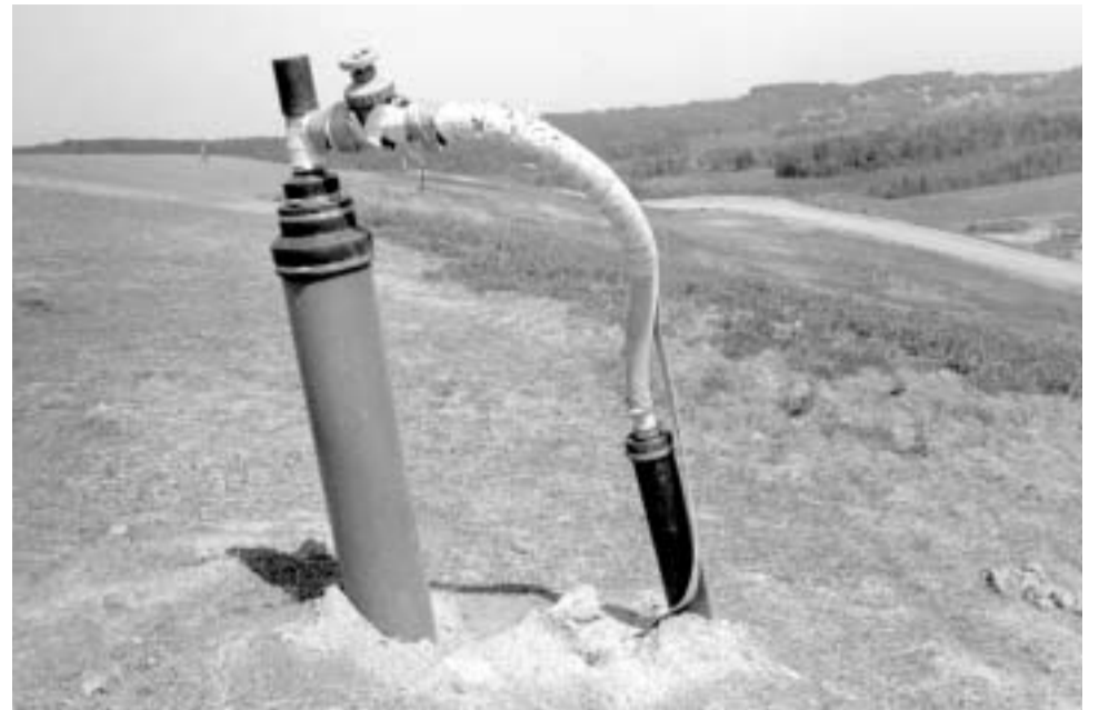
One of several wellheads at New England Waste Services' Coventry facility, which enable technicians to monitor the flow of gases and liquids within the landfill.
