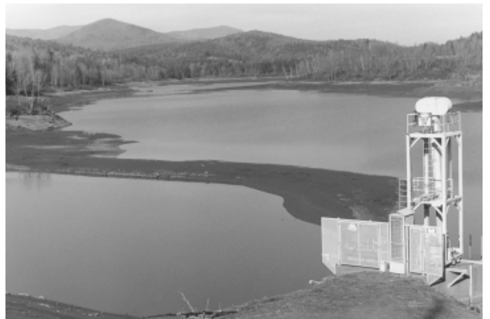
High and dry. The Wrightsville Reservoir is down to sand and puddles in this November photo. WEC drained the basin to aid in a police investigation.
