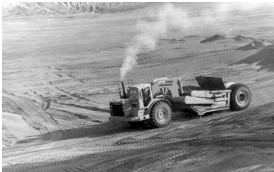
Site work began in November for a new 350-bed correctional facility in Springfield (above). The prison will use a modern co-generation system for electricity and heat, saving significantly on the state's power bill.
