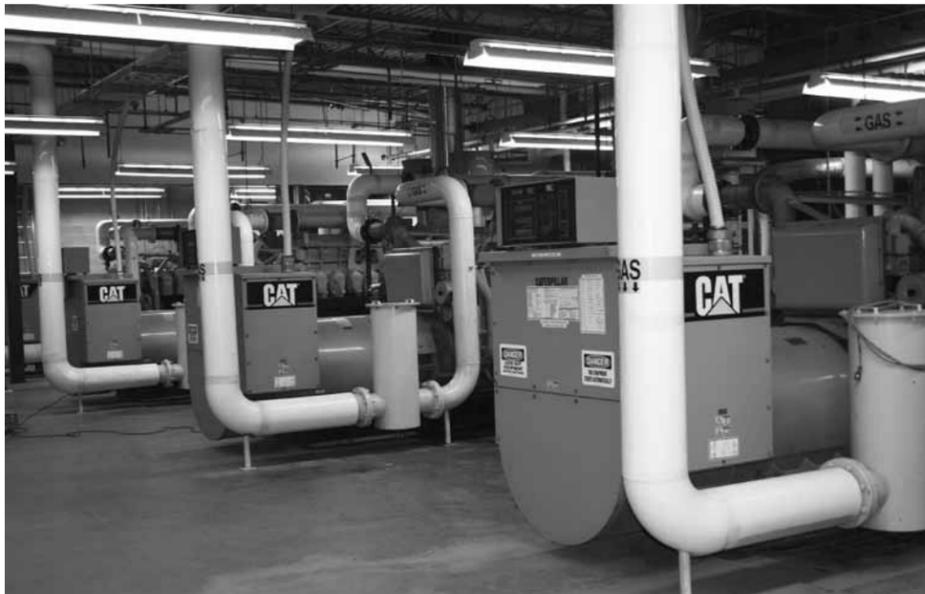
The engine room at Washington Electric's generating plant at Coventry. WEC has expanded to five engines to take advantage of the landfill's growing methane-gas production.
