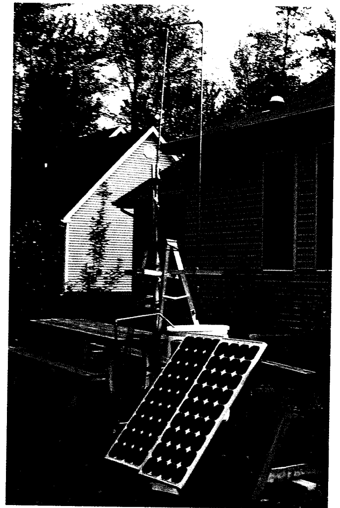
A backyard test determined that the PV-powered DC pump could provide adequate vertical lift for the drainback system.
