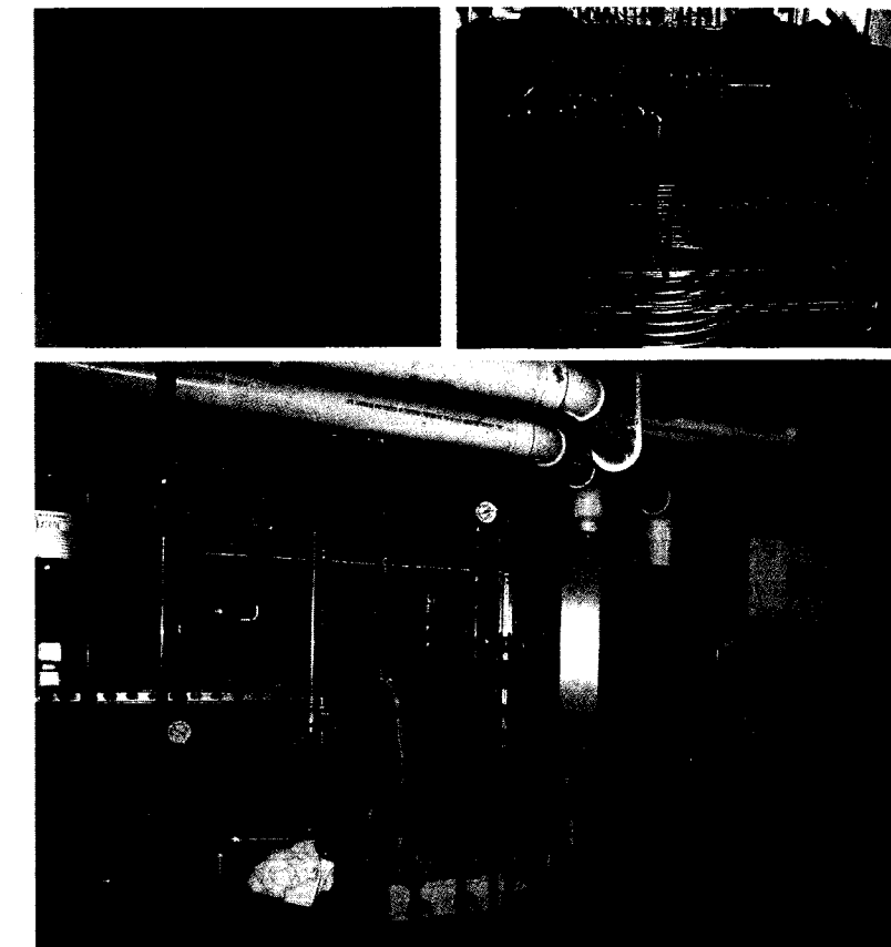
The concrete tank in the basement used for hot water storage. Right: Heat exchanger coils inside the tank. Below: The systems' mechanics wall, with the expansion tank, circulators, and boiler next to the PV system inverter and other electrical equipment.
