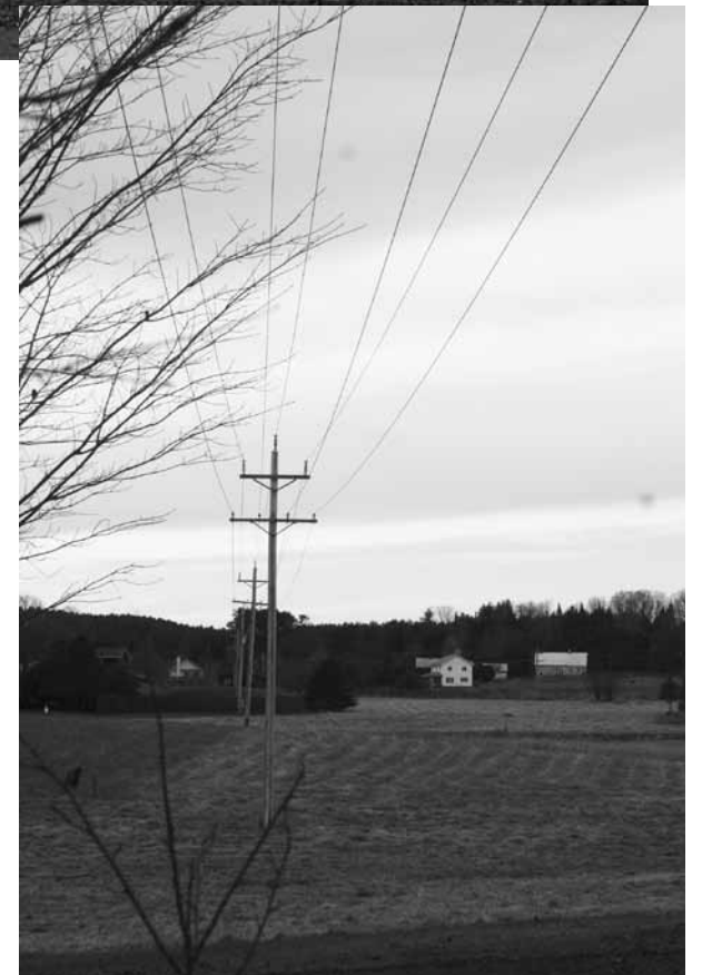
WEC's East Montpelier substation was dismantled this summer and replaced with a sturdier facility (above) offering better working conditions for staff, better environmental features, and the state-of-the-art equipment that enabled the connection at Pole #257 in Orange. At right: This is a “feeder” – three-phase power lines departing the East Montpelier substation and carrying lower-voltage electricity to a community of WEC members.
