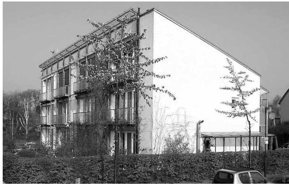
The term "Passivhaus" applies to an originally German construction design for buildings that use virtually no energy for space heating or cooling. This photo shows one of the first Passivhaus buildings, constructed in 1990. It is located in Darmstadt.
