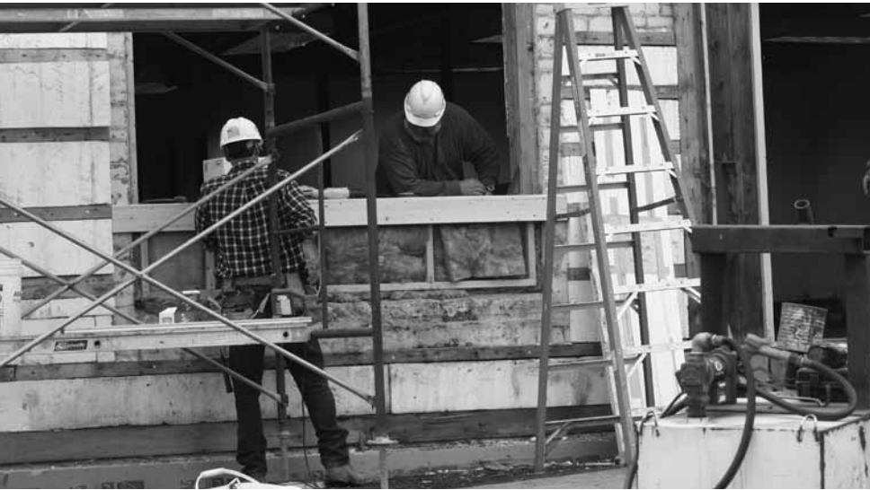
November 16 was a warm autumn day, which was a good thing because it gave contractors time to frame in the Co-op’s new windows before winter set in (above).
