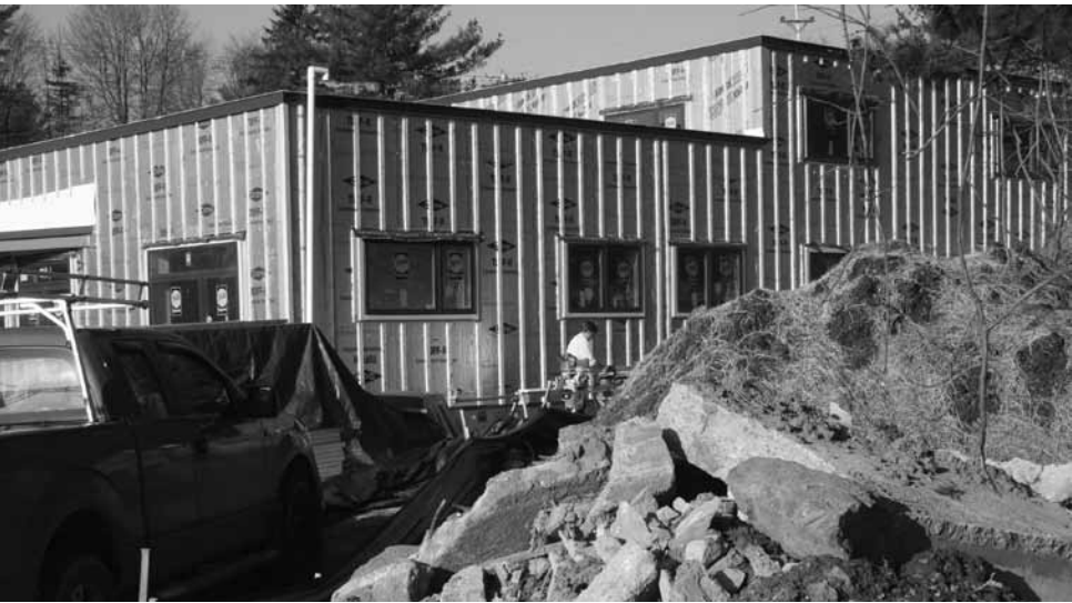
On March 21, 2012, contractors were excavating around the north wall of the building to construct a new drainage system.
