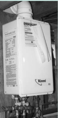
A wall-mounted, tankless, LP-fired water heater. This item, in the Mason-Sherwood home in Corinth, has cut their power bill more than in half. Their page 1 story continues inside.
