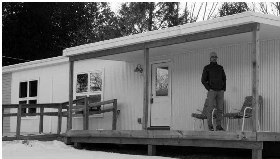
EVT’s Peter Schneider on the front deck of the VERMOD demonstration unit in Shelburne. Three residents of the mobile home park have already replaced their former dwellings with VERMODs, which adapt easily to the lot size and the footprint of conventional mobile homes.
