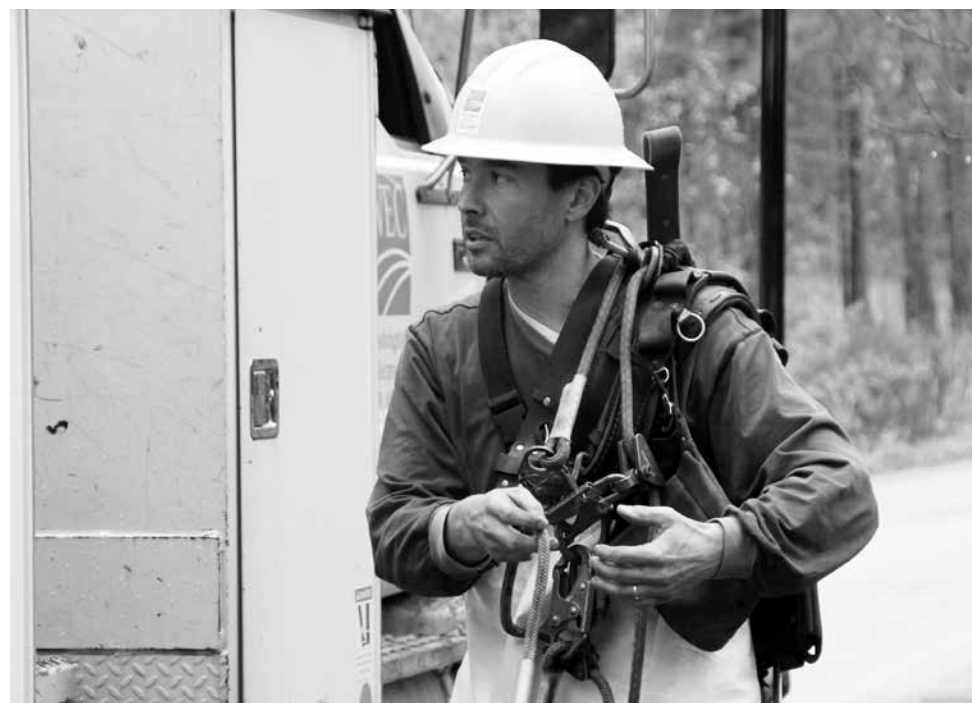
Kyle Sands repairing WEC lines during the October windstorm. He left to volunteer for hurricane recovery a few days after this picture was taken.
