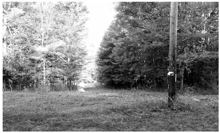
A cleared right-of-way prevents trees from falling on wires and allows operations crews to easily see and access poles, making restoration and repair safer and faster. WEC uses no herbicides to clear rights-of-way.
