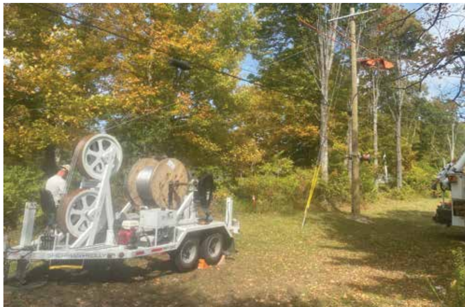
Line crew workers from WEC and contractor Riggs Distler work to pull messenger wire for the rebuilt lines along Bliss Road near Green Road in East Montpelier. The line is being rebuilt using Hendrix Spacer Cable system and other techniques to make it less susceptible to outages caused by storms and trees and is being funded in large part through federal grant dollars.
