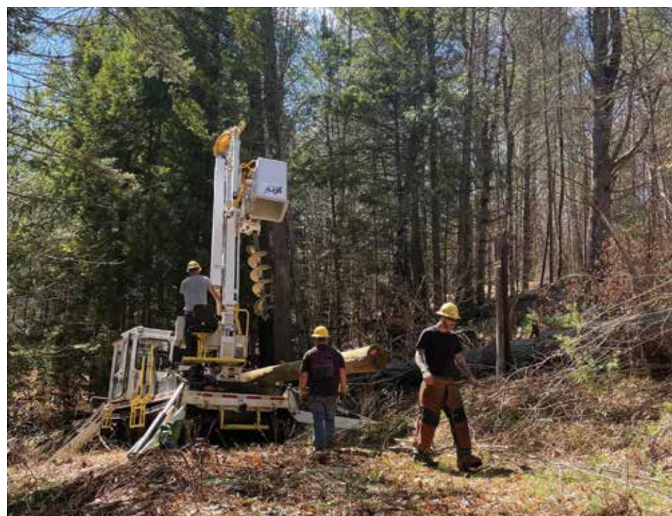
Line crew members replace a pole in Williamstown after an April tornado caused a surprise outage.
